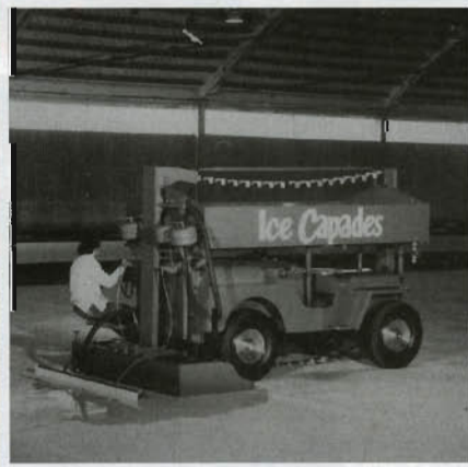
Frank Zamboni built the first ice resurfacing machine in 1949 for use at the Iceland Skating Rink in Paramount, Calif. The rink is still in operation today, just blocks from the Zamboni factory.
